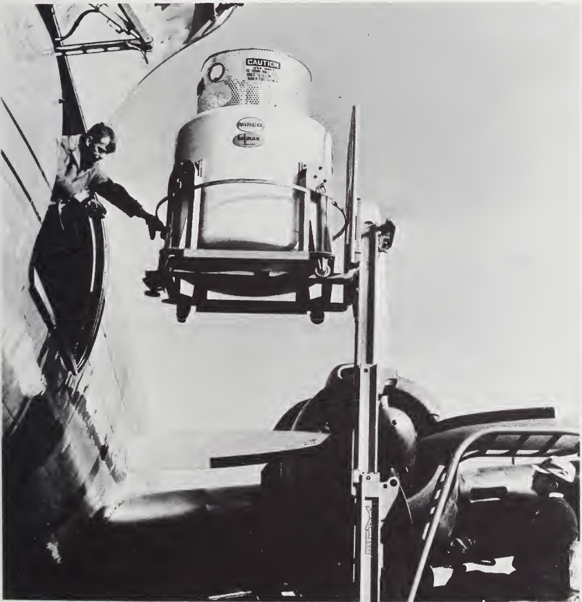
FIGURE 6.4. 500-l liquid helium container. (Courtesy of Air Reduction Co.).
